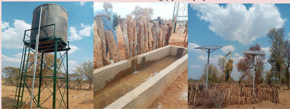
Solar powered borehole and irrigation system installed in ward 1, 5 and 6 in Tsholotsho District
