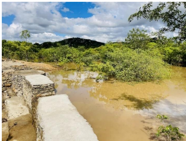
Gupiti dam in Mutoko
