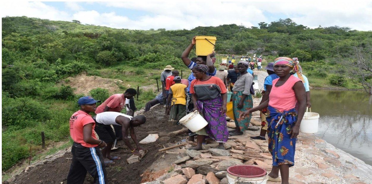
Weir dam construction in Rushinga District
