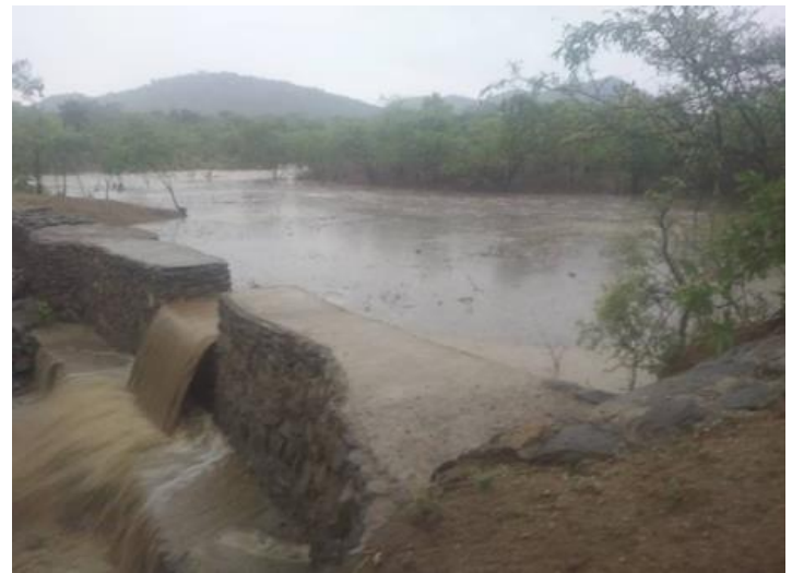
Gupiti weir dam at full capacity
