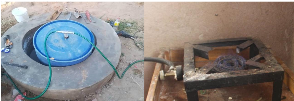
(L) Gas tank and (R) 1 plate stove installed in Mutoko.
